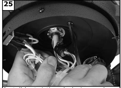
25 Install by twisting clockwise, replace screw removed from motor plate. Tighten all 3 screws securely.
